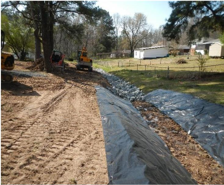
Severely eroded sections of a drainageway (left side images) were stabilized by widening and reshaping the banks. Woodchips and expanded media were placed in the bed of the drainageway, and covered with stone. These modifications have reduced pollutant transport by more than 30%.
