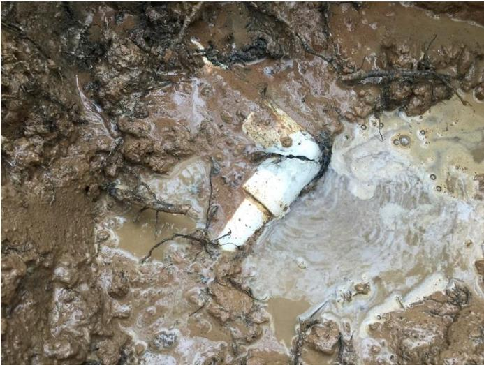
Malfunctioning septic systems were located and repair options considered. One property with a pump system, had a cracked supply line that was discharging effluent to the surface, and the runoff was reaching a nearby creek. The supply line was repaired.
