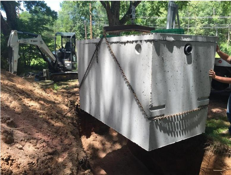
A new drainfield and septic tank were installed on properties with malfunctioning systems after repair permits were issued for the two sites.
